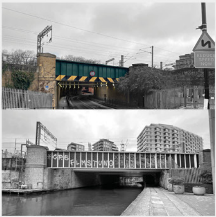
Local Precedent Railway Trusses and OHLE Catenary
