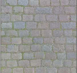
New Granite Setts Permeable as part of the SUDs
