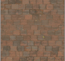
Brick Pavers Permeable as part of the SUDs
