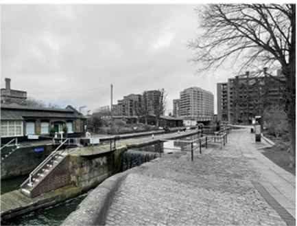
View 7 — Lock Cottage and Lock no. 4
