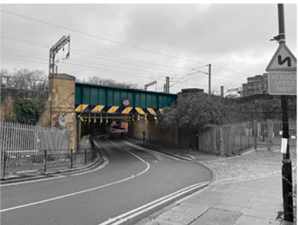
View 2 — South-East Underpass
