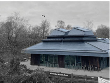
View 5 — CSNR from Coal Drops Yard
