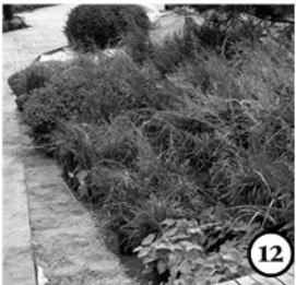
GREEN ROOFS Figure 3.2 Precedent Specification: Semi-Intensive 150–200 mm Substrate 15–20 species/sqm
