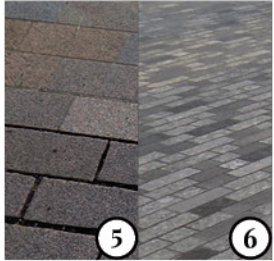
GRANITE STONE SETTS Spec.: Bush Hammered Colour: Pink and Mixed (Blue-Grey) Dim.: 100 x 100 x 200–300 mm Mortar: 10 mm
