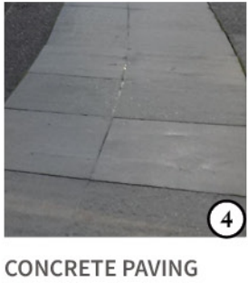
CONCRETE PAVING Spec.: Protects the HV Line Colour: Grey Dim.: 80 x 200 x 300 mm Mortar: 6 mm
